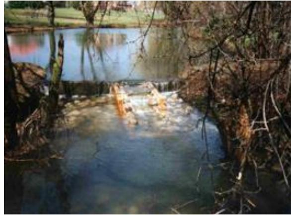
Small Step-pool fishway to allow passage by fish over a dam
