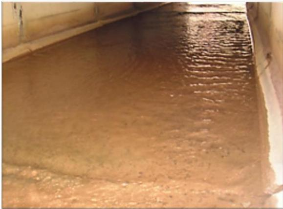
Shallow water in this perched culvert prevented the movement of fish upstream
