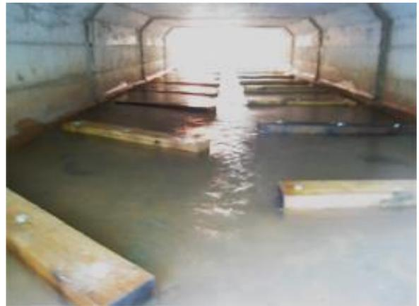
Baffle system installed in a culvert to increase water depth and provide fish passage
