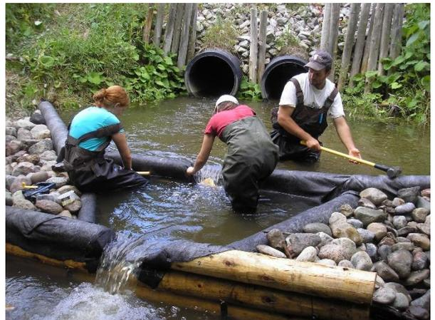
Perched Culverts mitigated by K-Dam Step Pool Fishway
