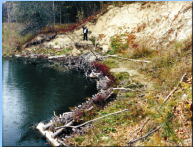
Figure 5.x: Native material revetment eventually fills in with sediment (top photo) and rapidly stabilizes with plant growth.
