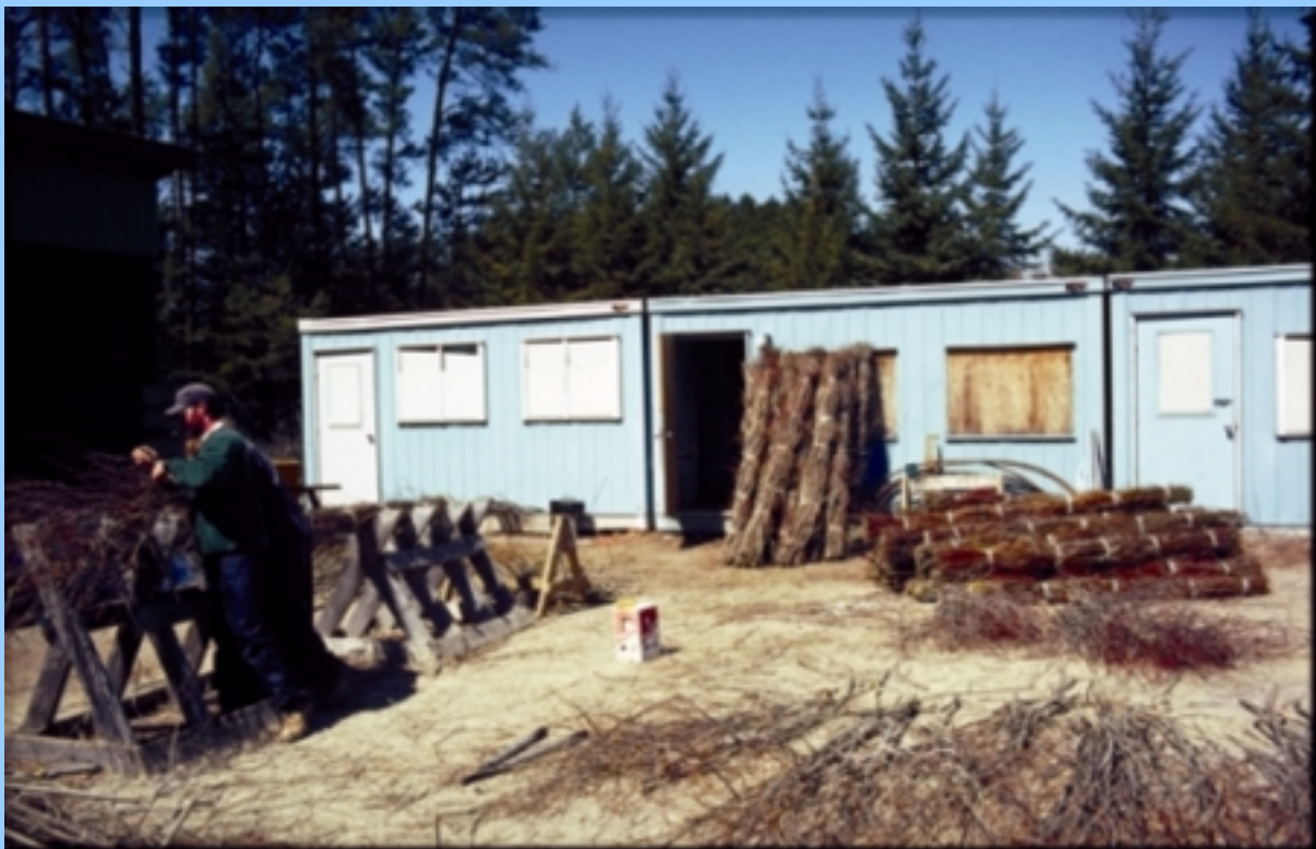
Figure 4: The use of a set of sawhorses makes it easier to tie the bundles. (photo by Rick Grillmayer)
