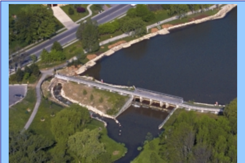
Where space is limited, a bypass channel may be restricted to only connecting the river with the impoundment. (Toogood Pond, Rouge Park photo)
