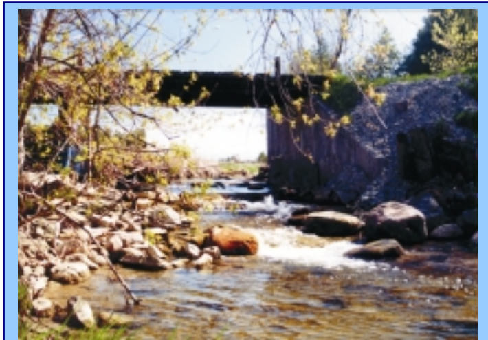
Partial removal of a barrier can restore some natural processes in a river.
