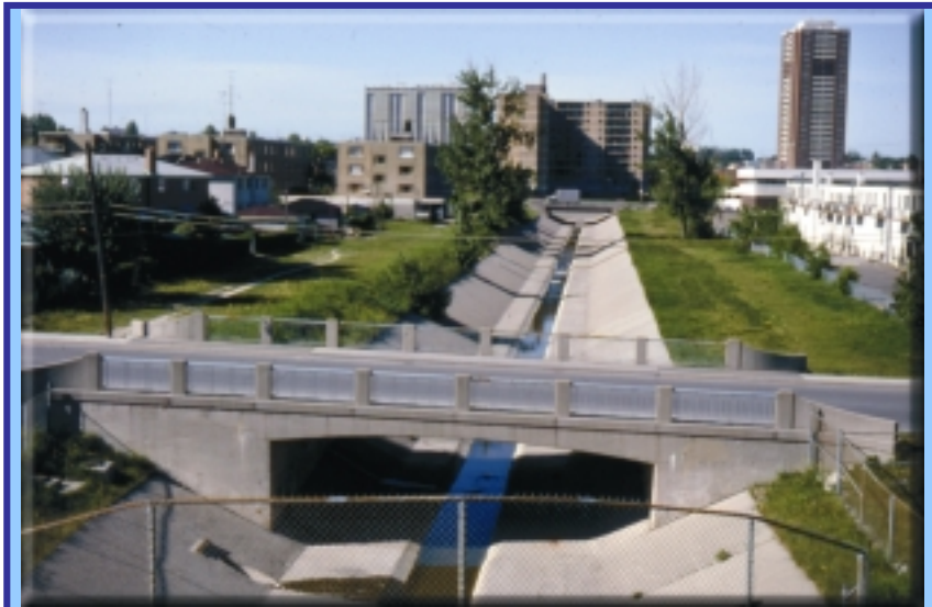
Figure 1.1: Many of our urban streams have been straightened and lined with concrete.
