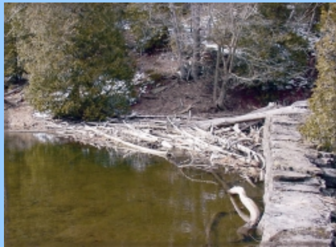
Dams block the downstream movement of sediment and large woody debris starving the downstream habitats of critical substrates.
