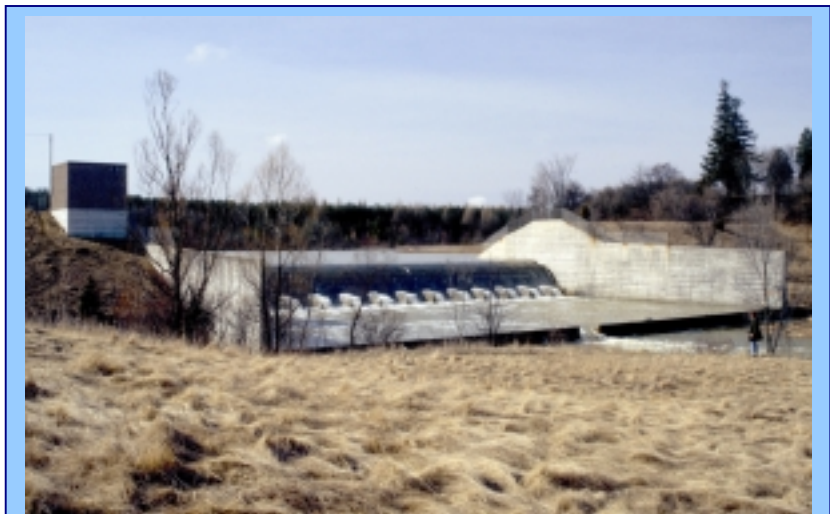
Dams and locks are structures that have the ability to control a volume of water behind them.
